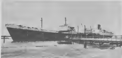
With the second phase of reconstruction work completed, the West Pier was placed back in service on December 24, 1971 as a safer and more permanent facility.
